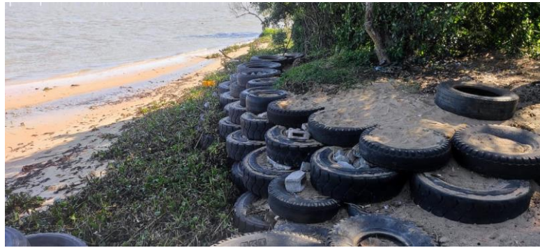
Figure 25: Tire used to protect against coastal erosion.
