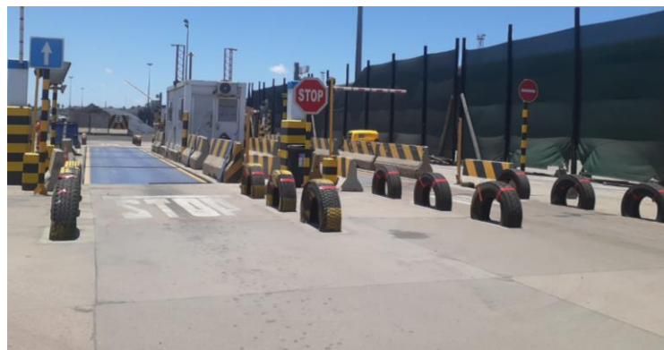
Figure 24: Tire used as flexible barrier in MPDC weighbridge
